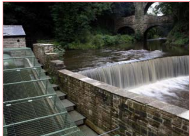
Torrs Hydro, in New Mills, Derbyshire, was the UK's first community owned hydropower scheme and has generated over 640,000 KWh of electricity since September 2008. Profits from the scheme fund a community grants programme.
